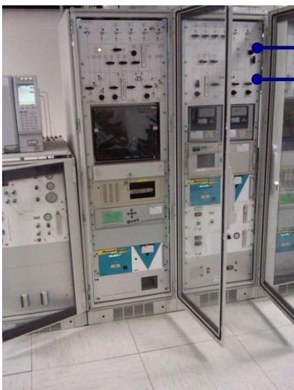
The system automatically transfer the product from field to laboratory, purge the tranfert line and flows sample to the
